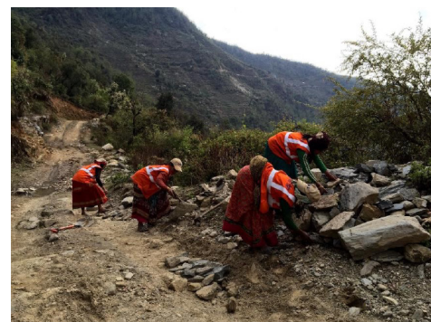
Beneficiaries within a Road Maintenance Group working along the road
