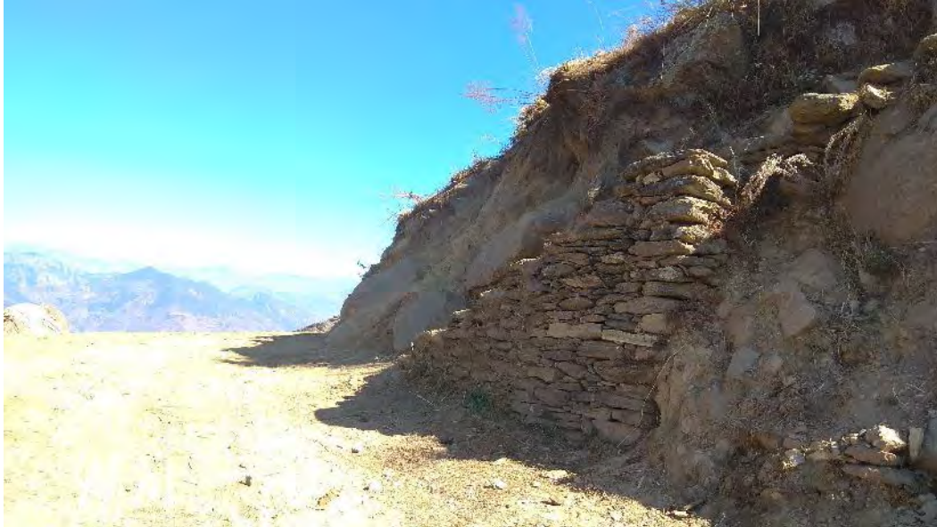
Photo 5: Chainage: 9+390. Foot trails constructed.
